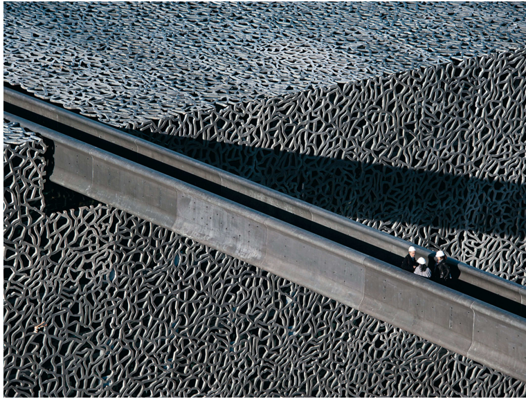
Figure 1.2.: Application of UHPC material in Museum of European and Mediterranean Civilisations, Marseille, French, photo from [2].
